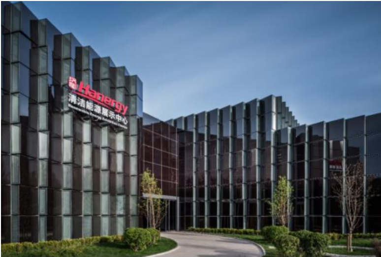
Peking – LEED Zero
