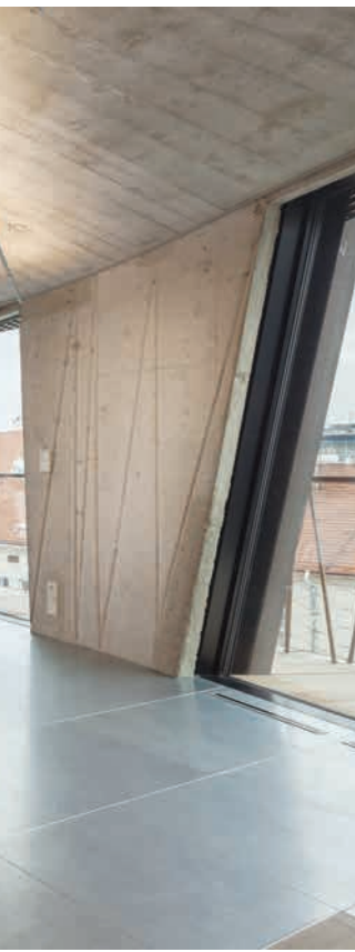
The Baroque Palace Špork in Hybernská Street, Prague, which was reconstructed in 1925 by Josef Gočár, has now been bestowed with a new spirit via a sensitive reconstruction by Stanislav Fiala.
